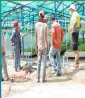
Working on installing the automatic irrigation
